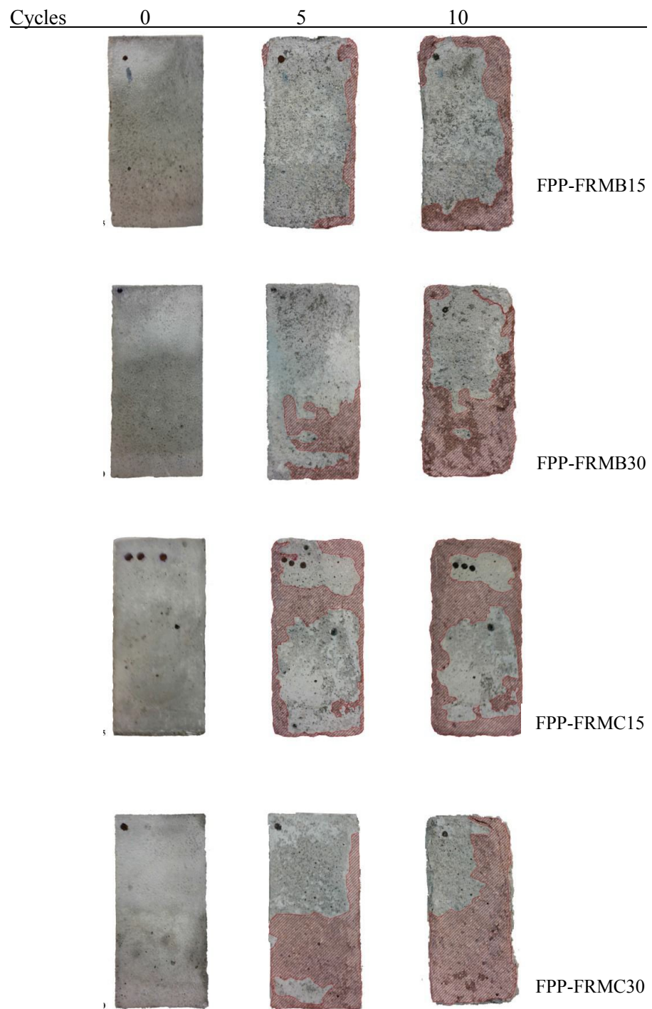
Figure IV.35 Comparison of the superficial degradation of FPP fiber reinforced mortars at different cycles
